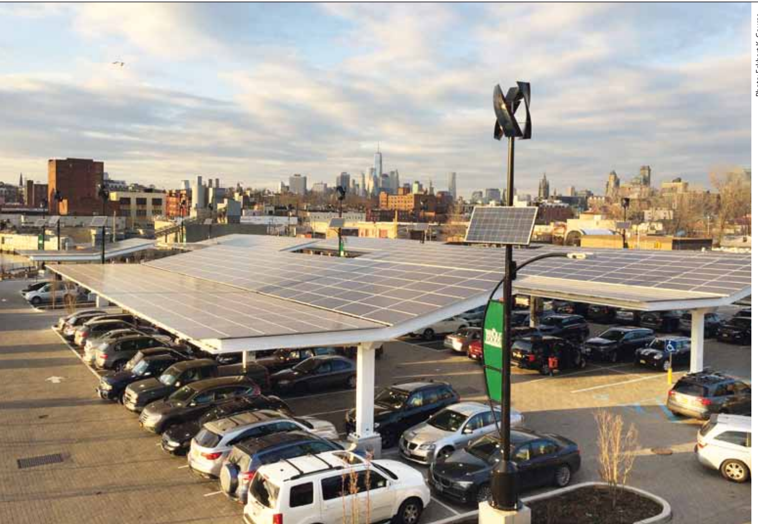
The U.S. commercial and industrial market segment comes in various shapes and sizes, like this 360 kW carport system in Brooklyn, New York City.
